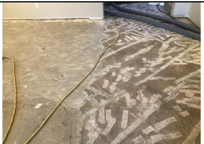
Photo 12: Example of concrete foundation slab area where tile was removed – grinder with HEPA attachment used on left side and not used yet on right side
