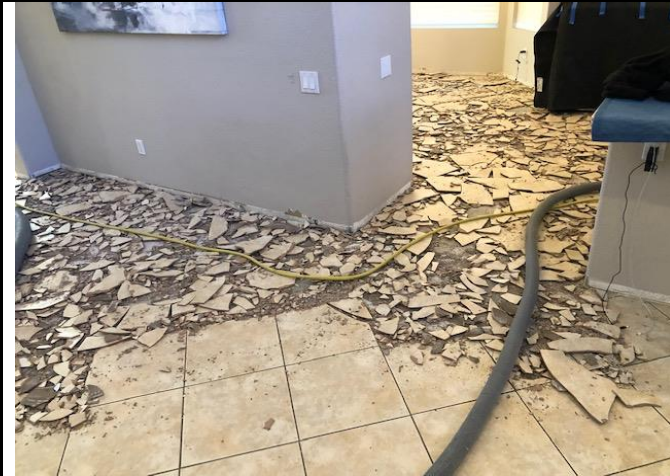
Photo 7: Example of large portion of tile/grout chipped up – debris to be removed and foundation ground to accept new flooring
