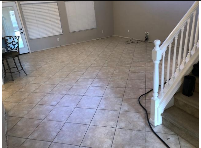
Photo 4: Overview of living area tile to be removed during project
