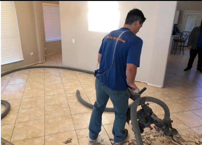
Photo 5: Example of employee fitted with personal pump and filter cassette while performing “chipping” operation with chipping tool and HEPA attachment
