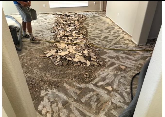
Photo 10: Example of rubberer collecting debris and placing into containers for removal
