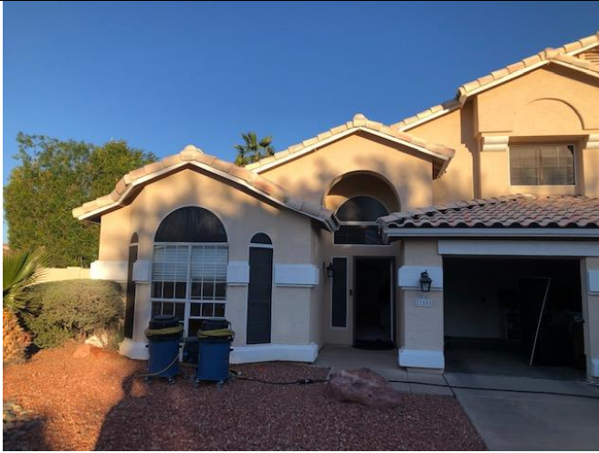
Photo 1: Work site - front
