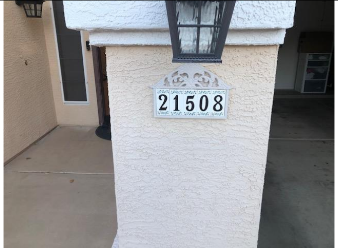
Photo 2: Work site address signage
